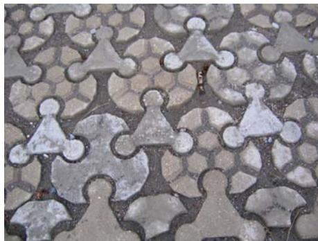
Figure 4. Hand laid interlocking pavers.
